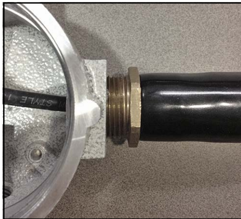
Figure 9: Torquing the Cable Gland
