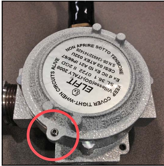
Figure 15: Set Screw of Junction Box
