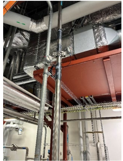
Fig. 2: Transducers with preamplifiers installed in one of the lines
