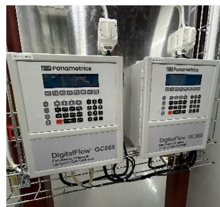
Fig. 1: 2 x GC868 measuring compressed air
