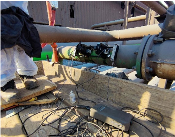
Pic. 2: PT900 & C-RR 1MHz transducers installed on short straight line
