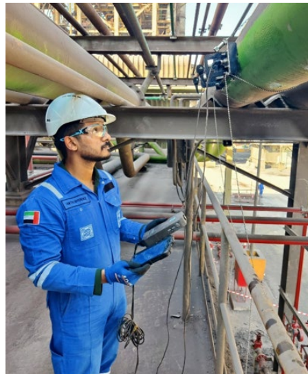
Pic. 4: PT900 & C-RR transducers (1MHz) on DN300 (12 inch) CS pipe
