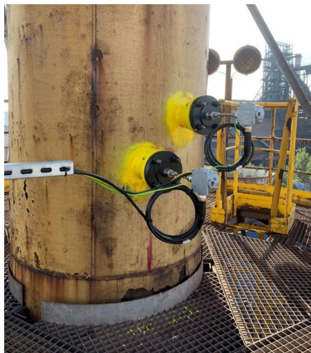
Picture 11. Combustion chimney with a T5 bias 90 setup on a DN1200 (48") pipe for blast furnace gas. Two applications from 2002 on raw coke oven gas DN1200 (48") and still working well.
