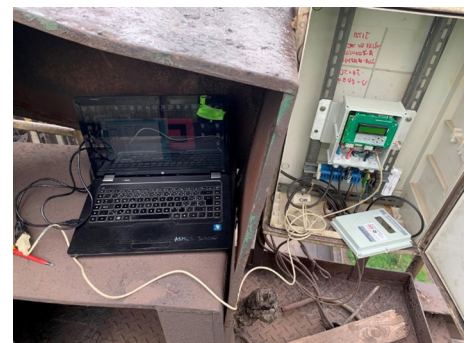
Picture 1: Replacement of AT868 flow meters on the Coke oven battery.
