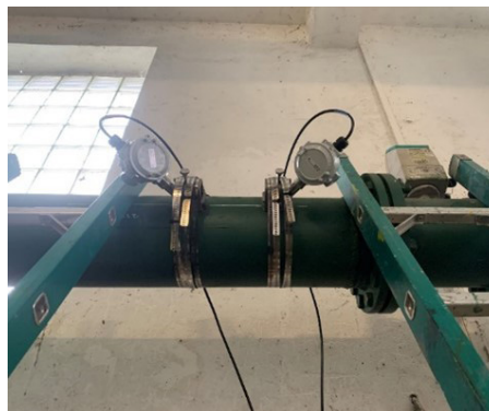
Picture 2. AT868 recently replaced by AT600 Clamp on C-RS installed from 2002 still works fine and kept in place.
