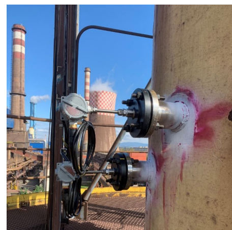
Picture 10. Combustion chimney with a T5 bias 90 setup on a DN800 (32") pipe for blast furnace gas.
