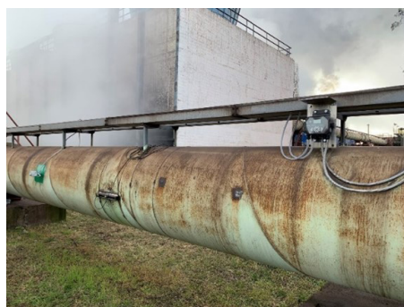
Picture 4. AT600 with WT wetted transducer solution from 1995
