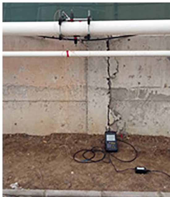
C-RS 401 transducer installation on the penstock
