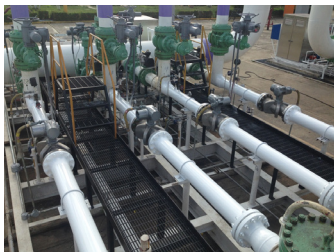
Sentinel LCT4 or LCT8 4 and 8 path liquid meters for applications 6 to 7
