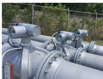
Sentinel LCT4 or LCT8 4 and 8 path liquid meters for applications 6 to 7
