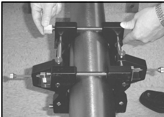
Figure 24: Installing Nuts onto the Fixture
