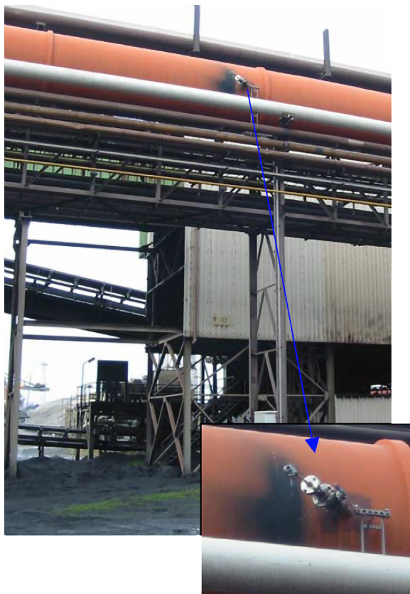
Fig. 2: Customer installation site
