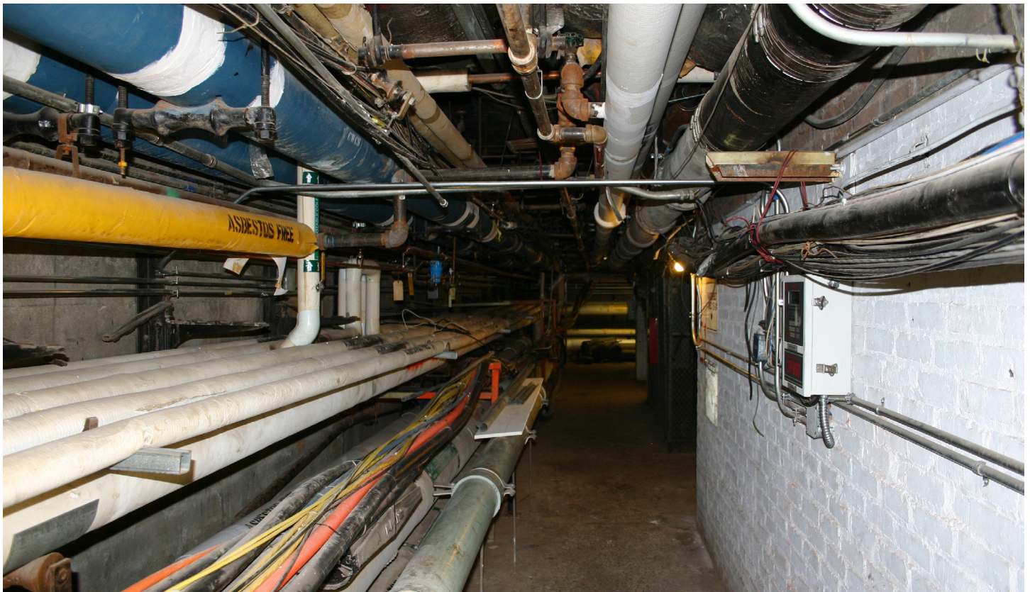
Figure 8. Energy measurement using an ultrasonic flow meter. (Photo courtesy of the University of New Hampshire)
