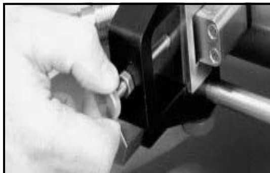
Figure 10: Installing the First Transducer
