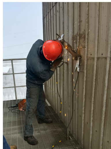
Fig. 1: Downstream nozzle installation
