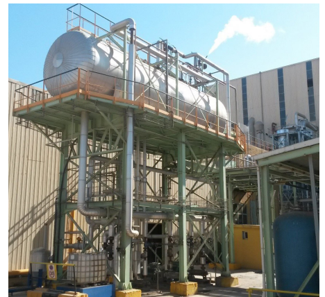
Condensate recovery vessel and downstream circuit of the condensates at the GRD-LaBelle plant
