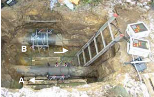
C-RL-304 (A) and 306 (B) transducers installed on pipe leading to and from the reducing station
