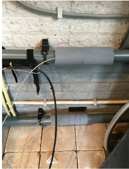
Both PT1000 elements insulated
